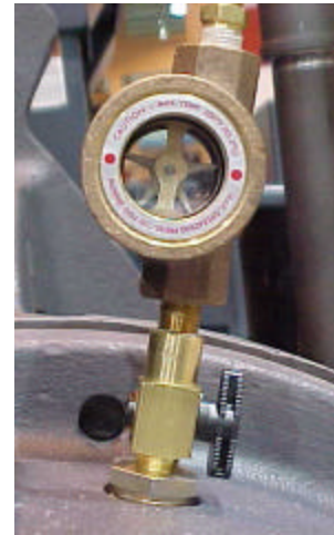
Figure 1.9 Visual indicator of water flow through vent lines
